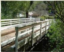
Meadow Way Bridge, over San Anselmo Creek, was constructed in the 1950's. The 70-foot long structure supports one narrow 10-foot wide traffic lane nearly 25 feet above the creek bed. The bridge spans an average to relatively wide section of San Anselmo Creek at a very sharp left channel bend, and serves as the only egress and ingress point to nearly two dozen residences across the creek from Cascade Drive.
