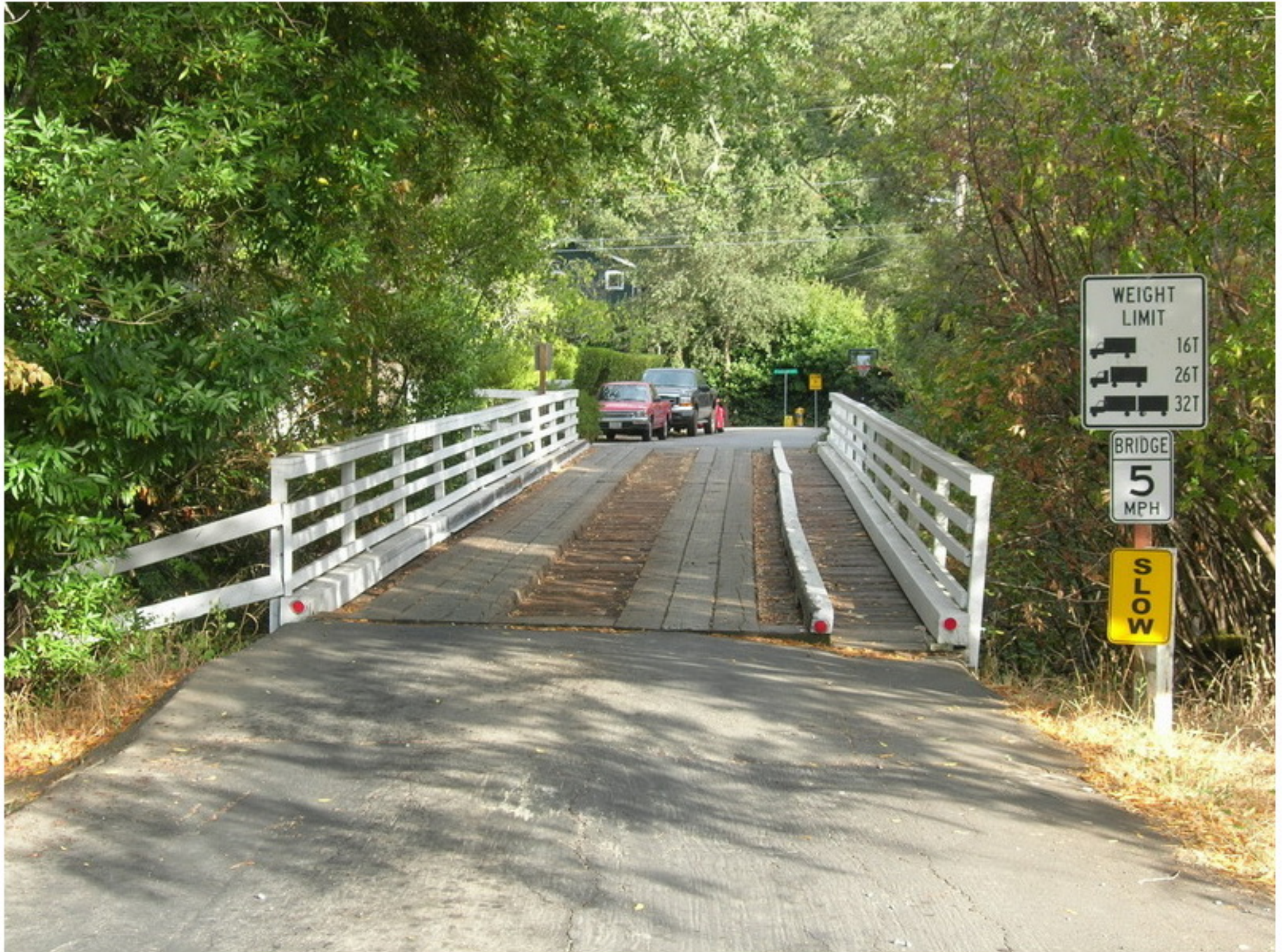
Photo No. 1 Roadway looking east.
