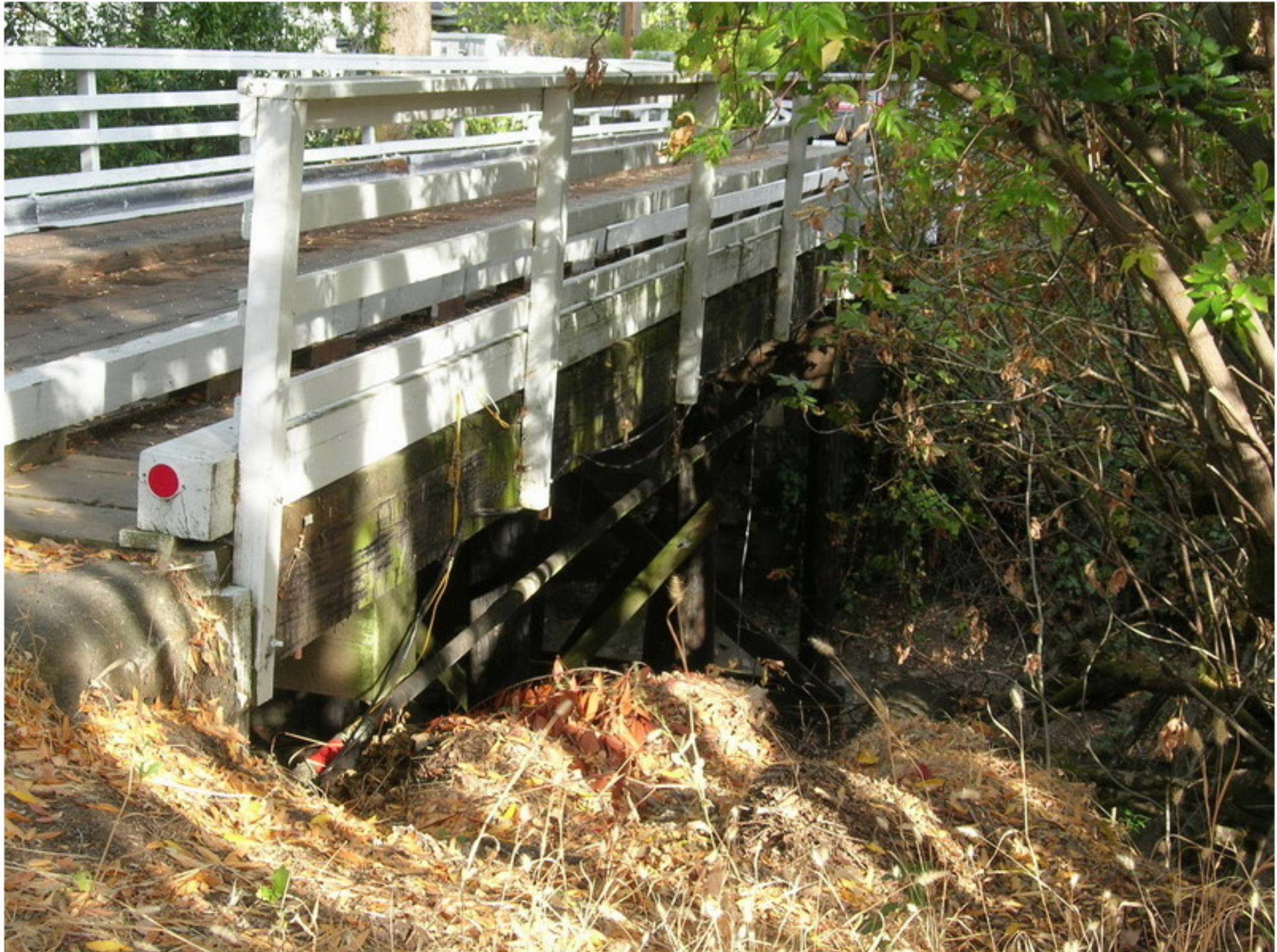
Photo No. 2 Elevation looking north.
