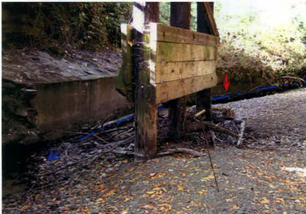
View upstream to right bank showing area of focused bed scour along the toe of the right bank and near Pier 4. The concrete toe wall bank protection structure at the outside bend channel position is undercut by as much as 4 horizontal feet
