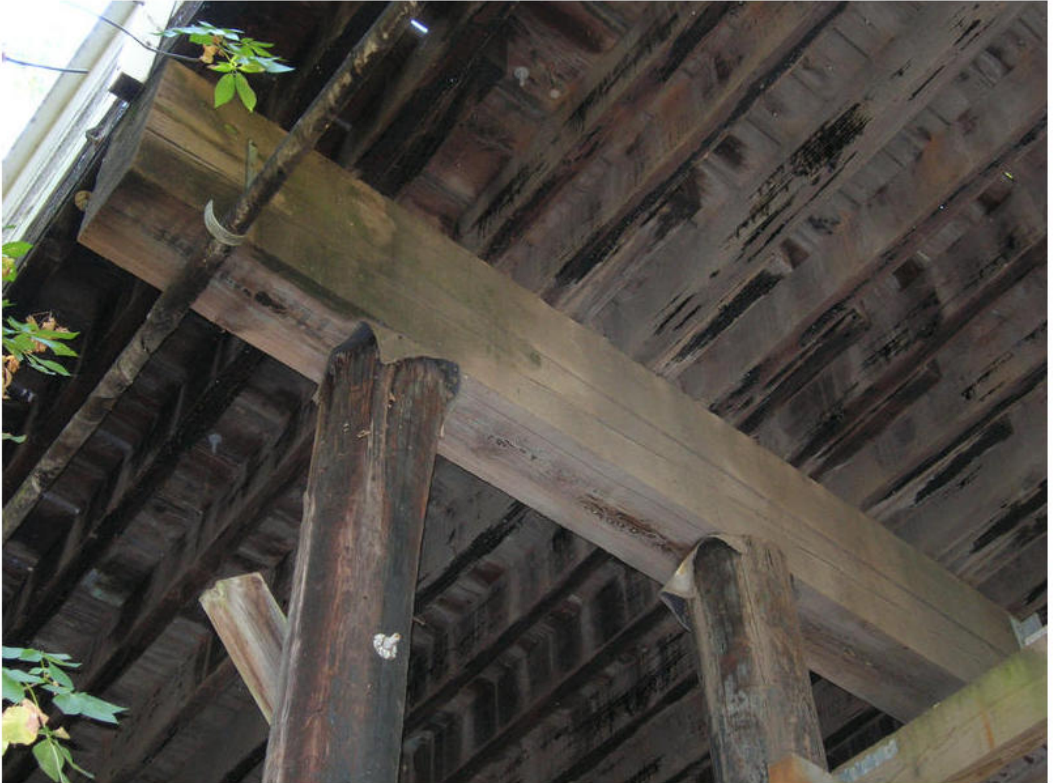
Photo No. 1 Horizontal check on Bent cap 4.
