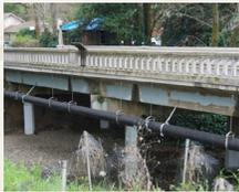
The Creek Road Bridge over San Anselmo Creek was constructed in 1929. It supports two narrow 10-foot wide lanes and narrow non-ADA compliant sidewalks on each side, and is supported on an abutment at each end of the bridge and on three sets of double columns in the creek. The Creek Road Bridge crosses a wide section of San Anselmo Creek and connects residents on Creek Road and Forrest Avenue with Bolinas Road, a main thoroughfare into downtown Fairfax.
