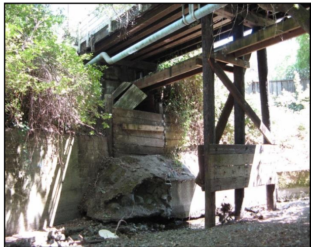
Meadow Way Bridge - Pier 4 (foreground) & Abutment 5 (back)
