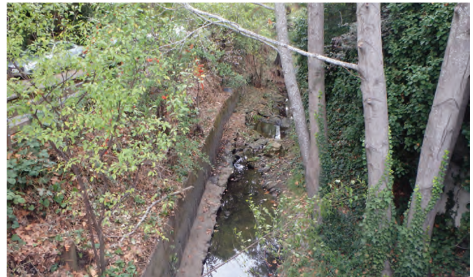
View 4. View looking northwest from Spruce Road Bridge.
