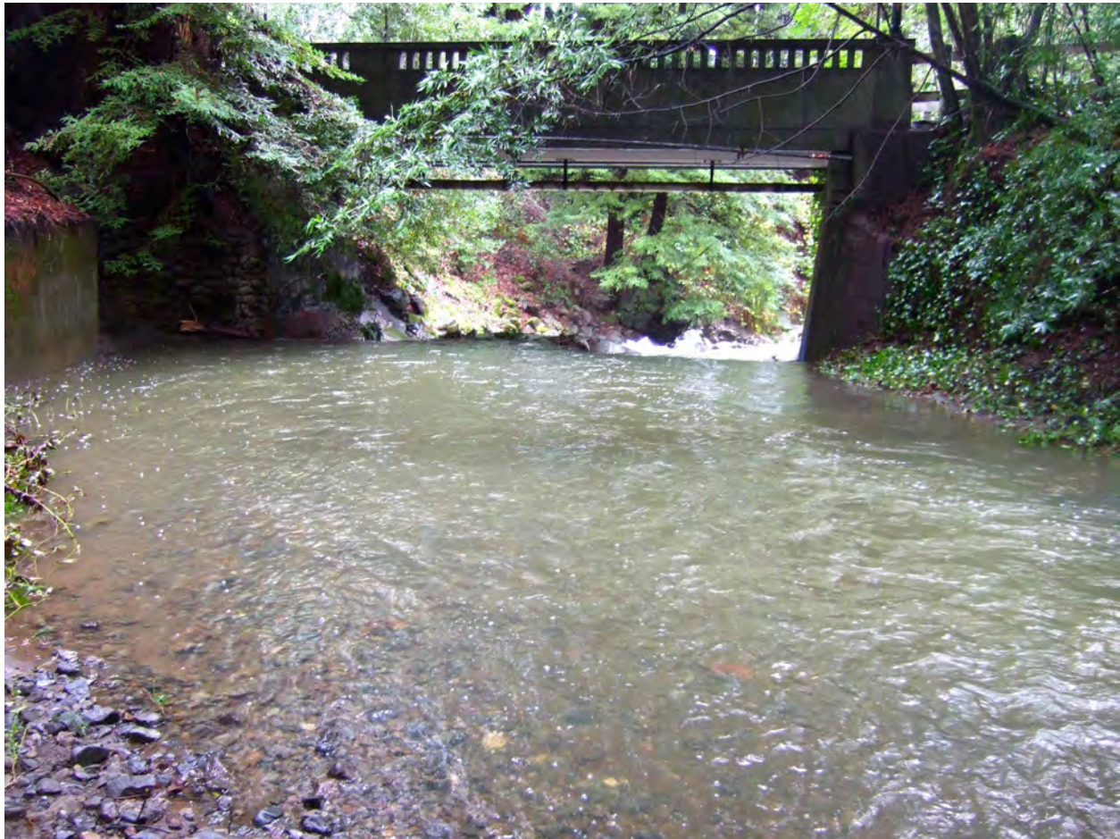
San Anselmo Creek Looking Downstream to Upstream Face of Canyon Road Bridge (December 19, 2014)
