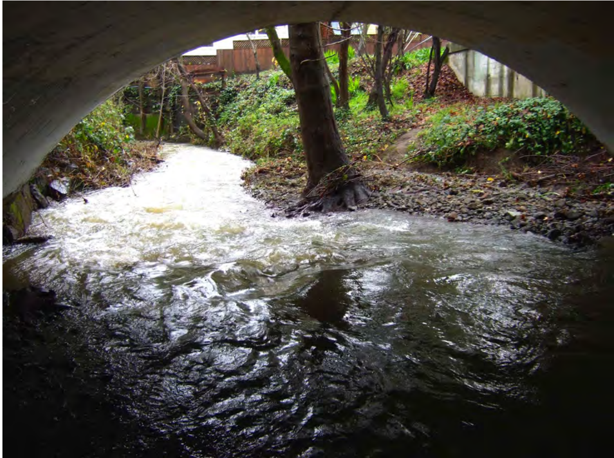
Looking Downstream to Fairfax Creek from the Upstream Face of Marin Road Bridge (December 19, 2014)
